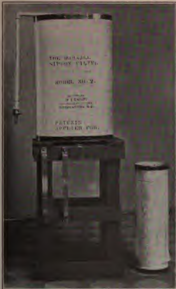
FIG. 59.—The Darnall filter, ready for operation.
